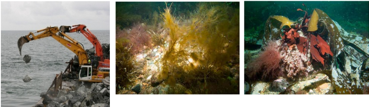
Plates 7, 8 and 9. Laeso Trindel artificial reef: construction of the reef (left) and benthic colonization on the reef boulders (from Dahl et al. , 2009).
